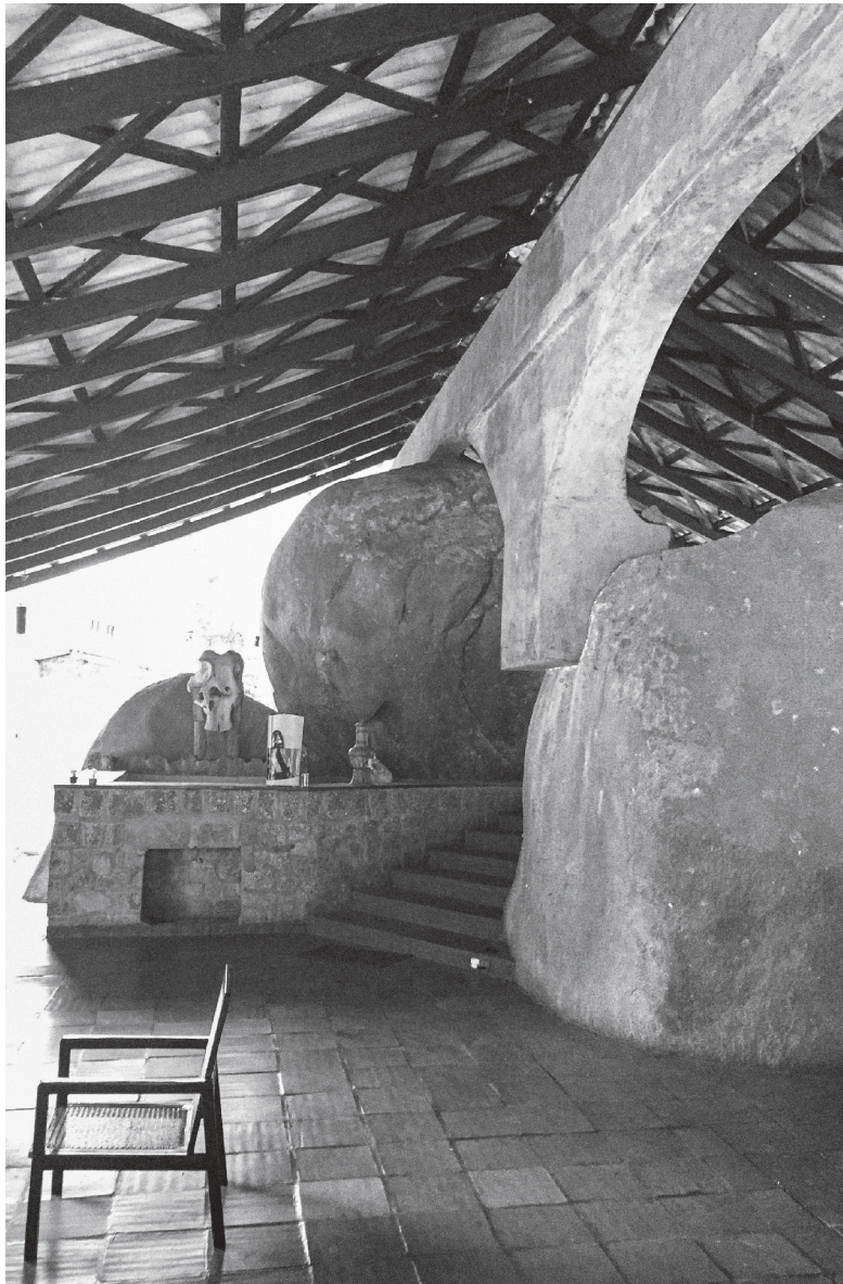
Above and right: The entry and living space of Geoffrey Bawa’s Polontalawa Estate Bungalow. The main roof structure is supported by boulders. Near Nikarawetiya, Sri Lanka, 1963–65.
