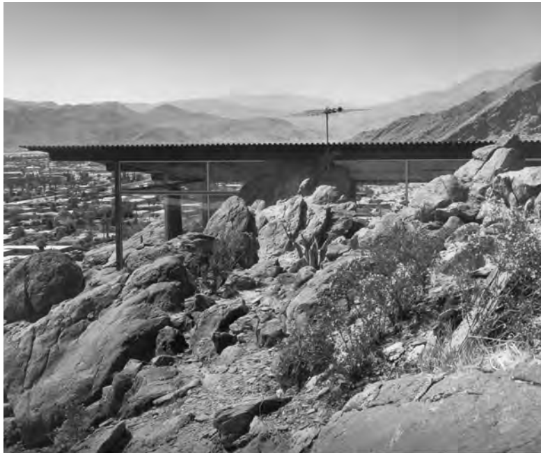
Above and right: At the Frey House, a boulder seems to interrupt, rather than support, the building's tent-like steel frame. Albert Frey, architect. Julius Shulman, photographer. Palm Springs, California, 1964.
