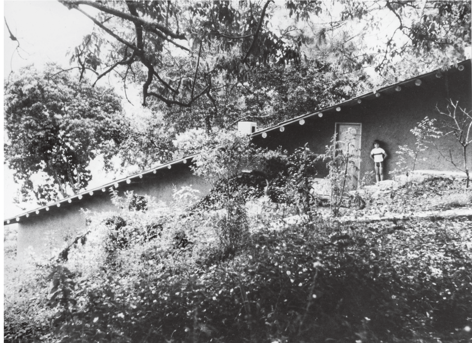
The roof as an abstraction of the existing topography, drawing a sharp diagonal line through the forest landscape. Ricardo Legorreta. Casa de Fin de Semana, Valle de Bravo, Mexico, 1973.
